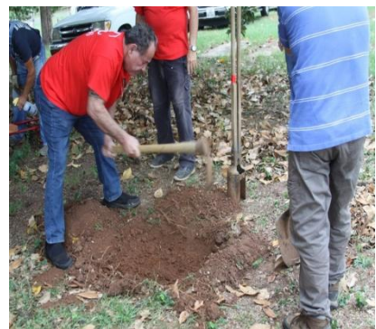
starting the dig
